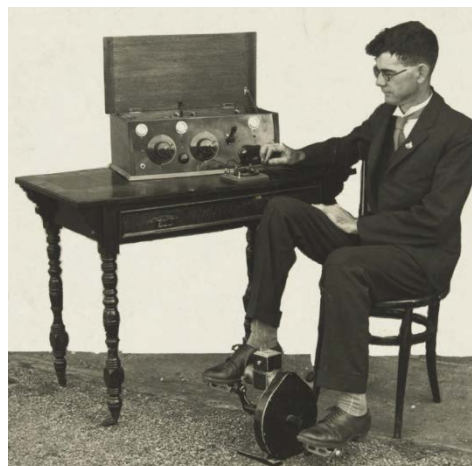
Mr. Alfred Traeger transmitting by a pedal-powered wireless, ca. 1929 National Library of Australia nla.obj-137929073
